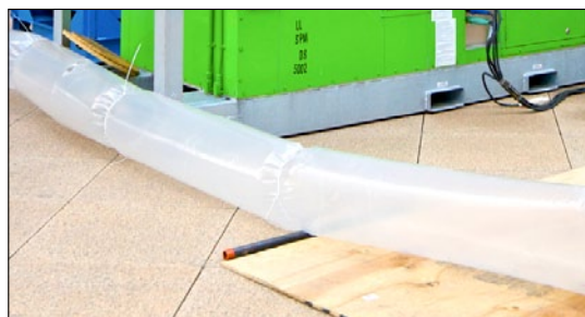
Lay-flat ducting in use
