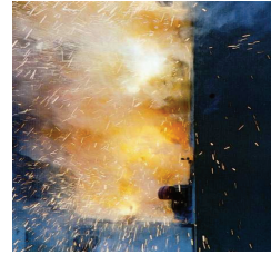
Photo courtesy of Schneider Electric
