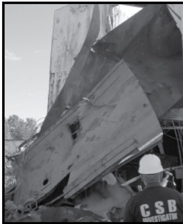
Figure #3: Blast containment structure damaged by steel blast panel
