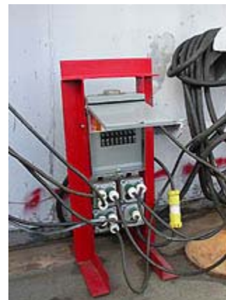
Circuit breakers in panel box can be used to deenergize circuits (and appropriately tagged) before working on the circuit.
